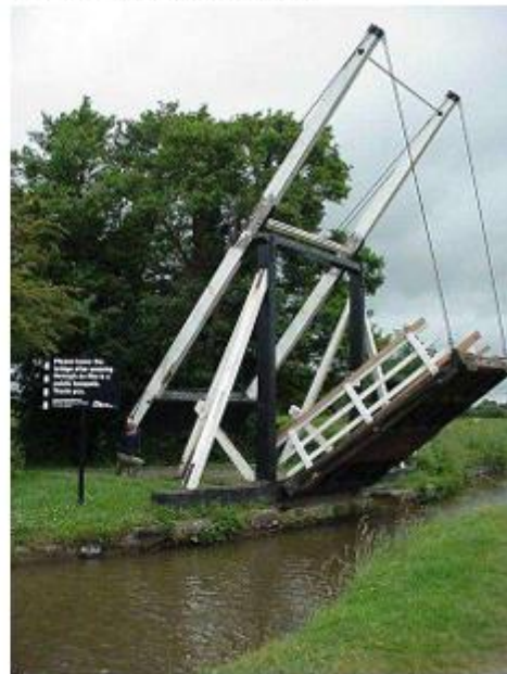
A canal lift bridge using levers to enable a person to raise a bridge so that a boat can pass along the canal
